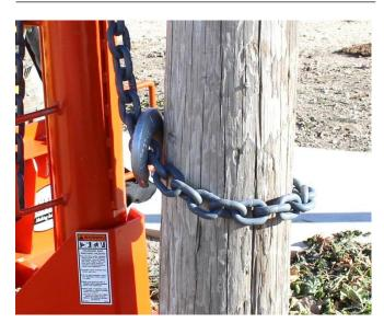
4) Wrap the chain/wire rope around the pole and secure the grab hook back on the chain/wire rope as shown above.
