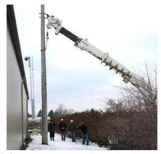
Secure the upper part of the pole with a digger derrick truck pole claw. Position the load securement chain above the balance point of the pole being pulled (see above).
